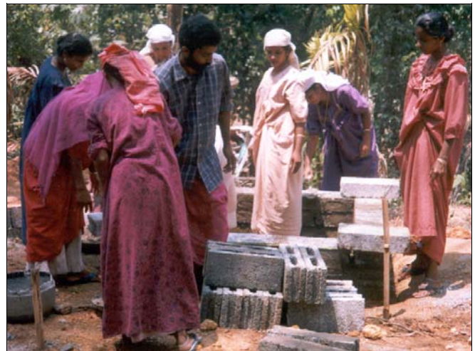
With the help of SAFF, 20 women from a local Sangham in Thamarassery, Kerala, India, construct sanitary double pit latrines under the supervision of an instructor.
